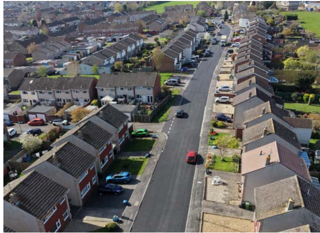
Lays Drive in Keynsham was among the first to benefit from the council's 2026 resurfacing programme in March
