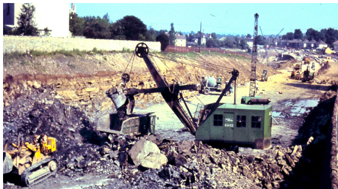
Marion Leitch on the bypass a few days before it opened Below, a face shovel excavating the cutting at Station Road Photos from the Russell Leitch collection
