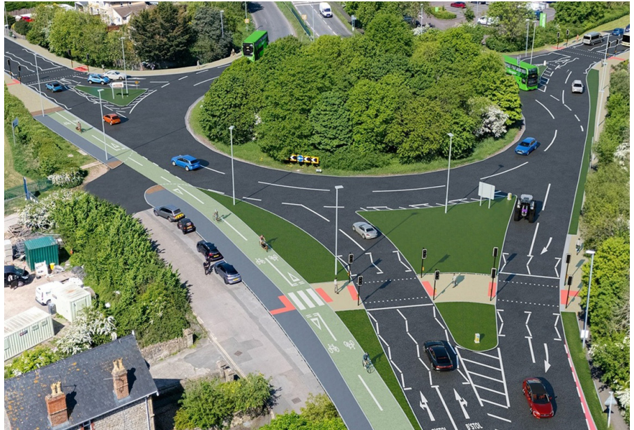
The Broadmead roundabout is to get three new crossings for pedestrians and cyclists
