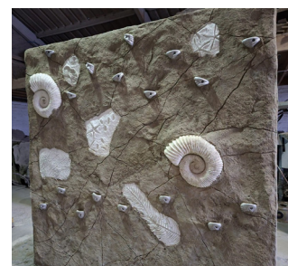
A climbing wall being built for the play area Photo: B&NES Council
